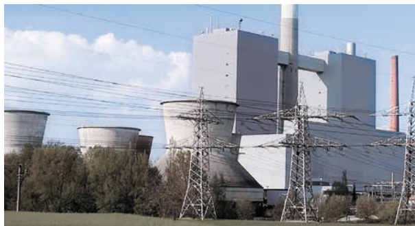
Indispensable for power plant
